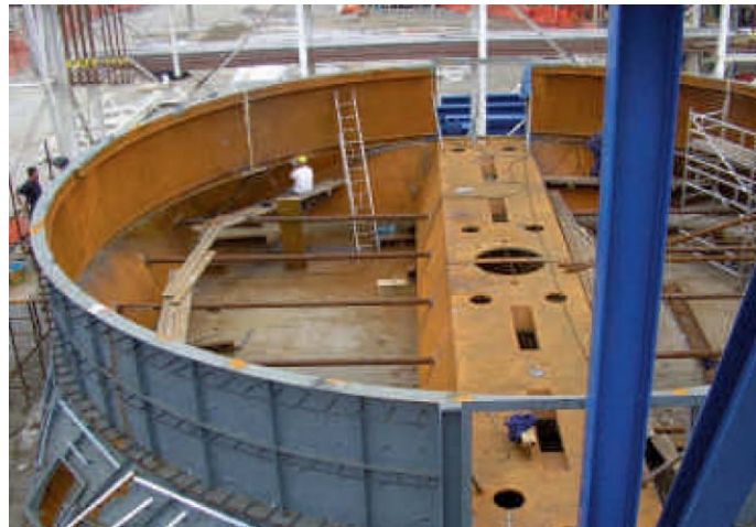
Regenerative Heat Exchangers with Stationary Heating Surfaces (ROTHEMÜHLE-Stator System)
